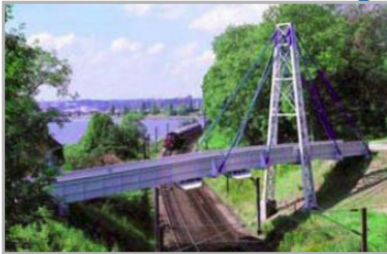
Pedestrian bridge in Denmark, 130 feet long (1997)
