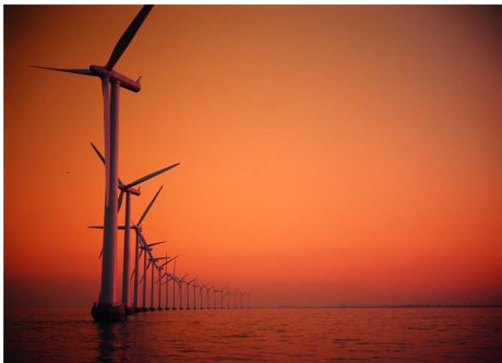
Each rotor blade is 36.8 m long. www.lmglassfiber.com
