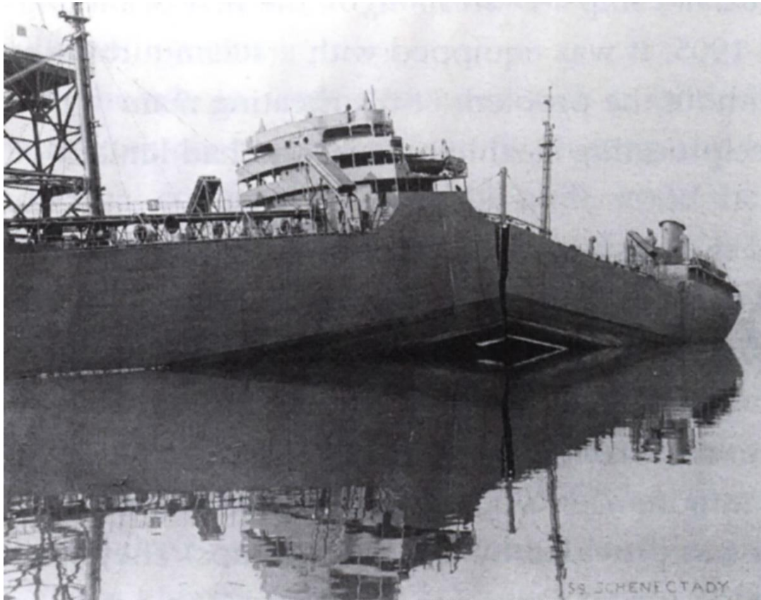
A liberty Tanker, 16 January 1943, split in two while moored in calm water.
