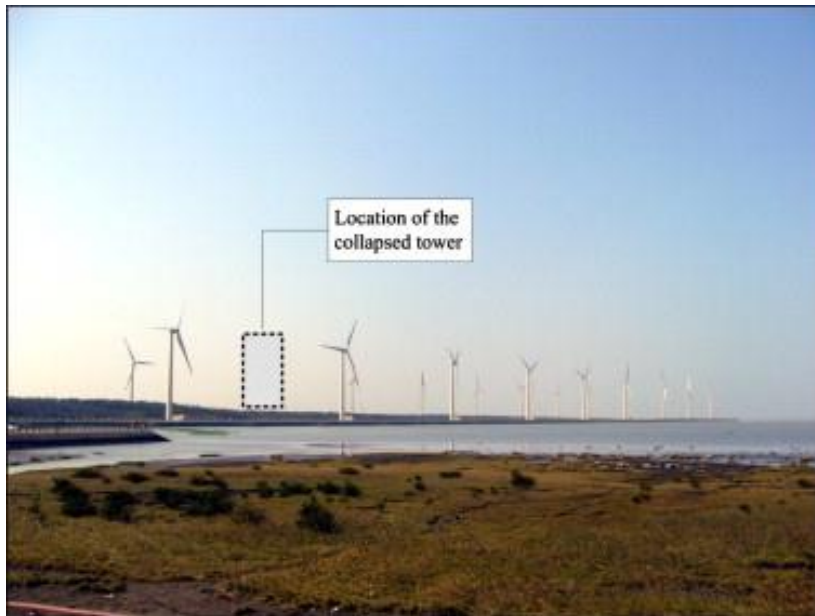
The current wind turbine field
